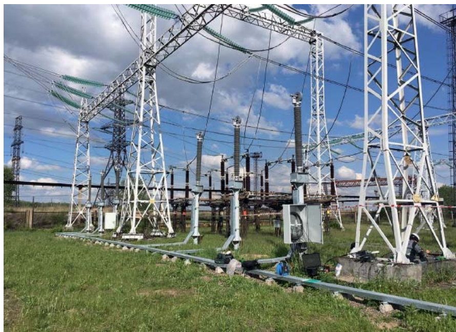
Figure 3. Columns with combined electronic optical current and voltage transformers 220 kV
