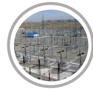
Transmission and distribution of electricity
